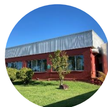
Tordera R&D Centre (スペイン)
